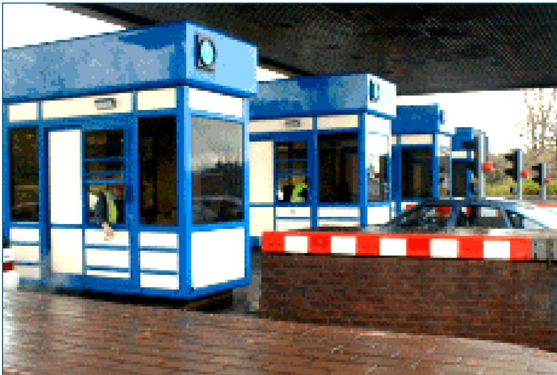
Figure 5: The River Itchen Bridge Toll Booths
